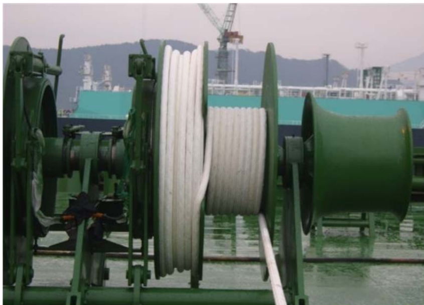
Figure 1.2: High modulus synthetic fibre mooring line on split drum winch
